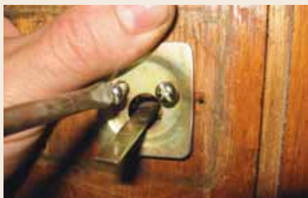
Insert the cylinder and attach the back plate
