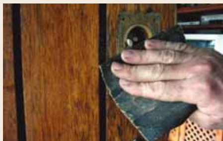
Give the area a light sand to remove debris and wood splinters
