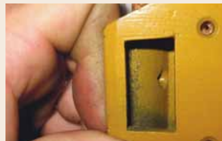
Once you've attached the lock on the inside door, fit the strike to the door jamb
