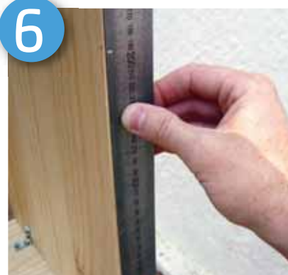
Mark off the positions of the internal shelf/shelves
