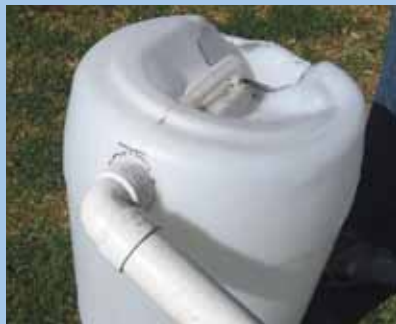
PVC piping angled to the side away from the barrel will direct overflow water away from your home's foundation
