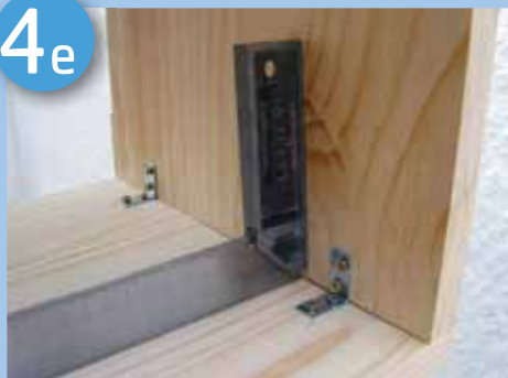
Check that the join is right angles with a set square
