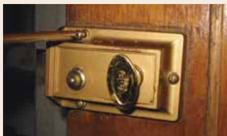
Use a screwdriver to remove the old lock
