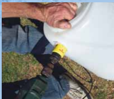
Drill out the overflow hole at the side of the barrel
